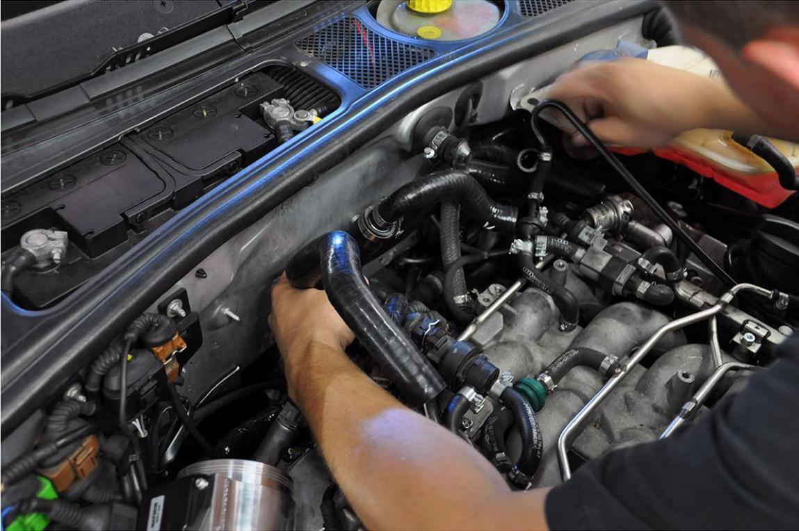
**Step 12** – Connect the vacuum hose to the N75 valve and clamp securely.
